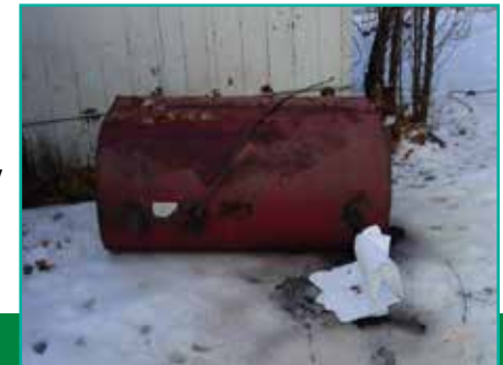
Overturned oil tank
